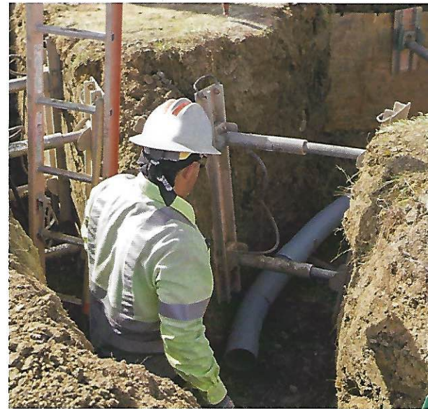
Julian Undergrounding Project
