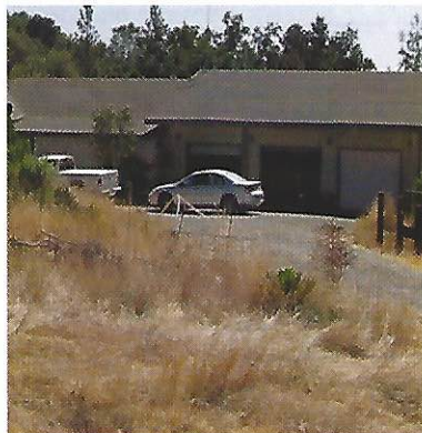
DEFENSIBLE SPACE NONCOMPLIANT
